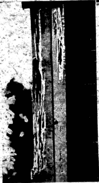
owing to lack of protection, the destruction caused by White Ants was so great in this structure as to render it useless in an incredibly short time.
