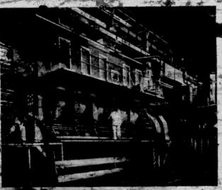
H & W 2 cycle Opposed Piston Engine Alternation Set 2270k Won test bed. One of two test for the Darles, with H & W Alternators or D.C. Generators of Messrs, Balfour, Beatty's Co., Ltd. consultants by
