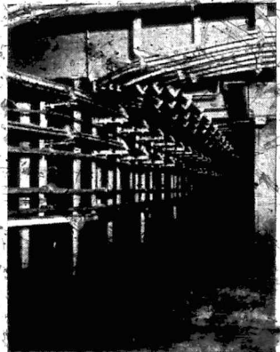
Central Electricity Authority. Main cable tunnel in Porthsmouth Power Station.
