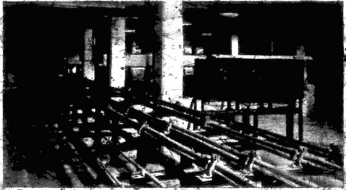
Electricity Authority of Cyprus. Cable basement in Dhekelia Power Station.
