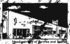
Headquarters of Service and Sales Organisation in Nairobi
