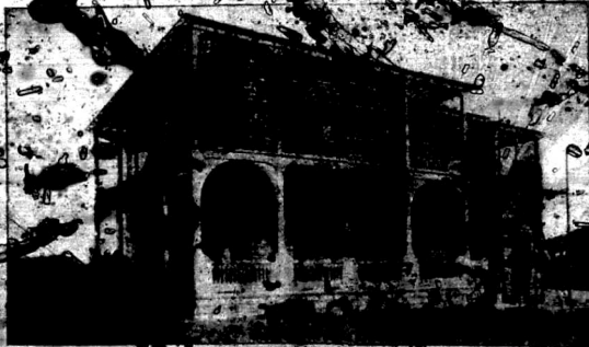
Sectional Building Erected in Tropical Africa
