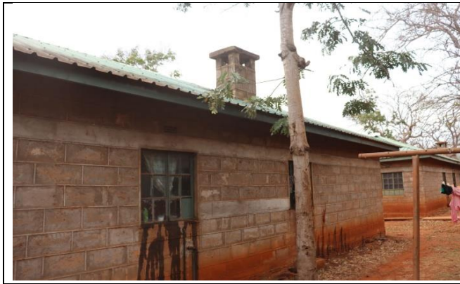
a. Residential building
