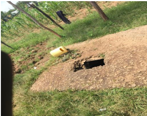
Figure 5: Groundwater source at high risk of contamination
