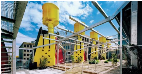
Fig 81 Image showing the wind turbines on the Council House Building 2
