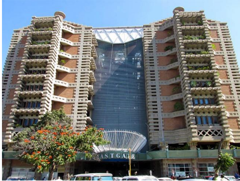
Fig. 97 Image showing Eastgate Harare. Source: Eastgate-Centre-in-Central-Harare-Zimbabwe.jpg (650×488) (eaconstructionsdigest.com), 2023
