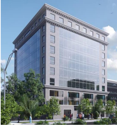
Figure 114 Image of Delta Chambers building, in Westlands, Nairobi. Source: R.9593f491a537ce360540a9f871ac82fd (750×450) (bing.com)
