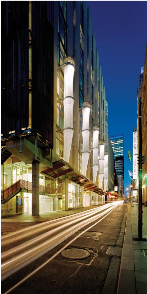
Fig. 78 Image showing the shower towers on the Council House building. Source: Fig. 5 image showing CH2 office interior.
