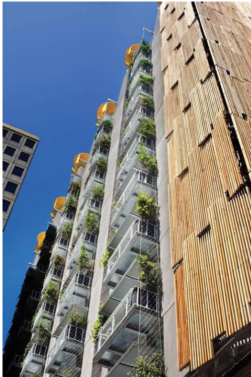
Figure 87 Image showing CH2 Building.
