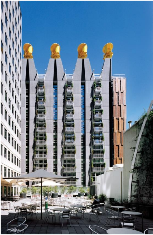
Fig. 75 Image showing the CH2 shower towers. Source: CH2 Melbourne City Council House 2 / DesignInc | ArchDaily, 2023
