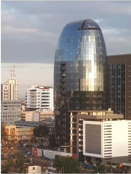
Figure 6 Image showing One Africa building in Nairobi.
