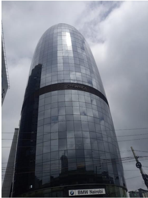
Figure 105 Image showing One Africa building tower. Source: Author, 2023
