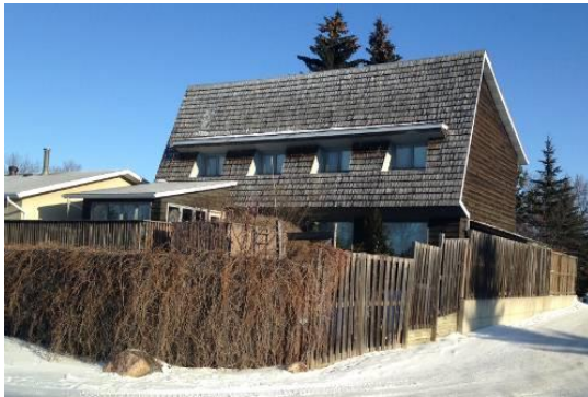
Figure 26 Image showing The Saskatchewan Conservation House " (1976). Source: saskatchewan_house_orr2_kleiner.jpg (499×333) ( passipedia.org )
