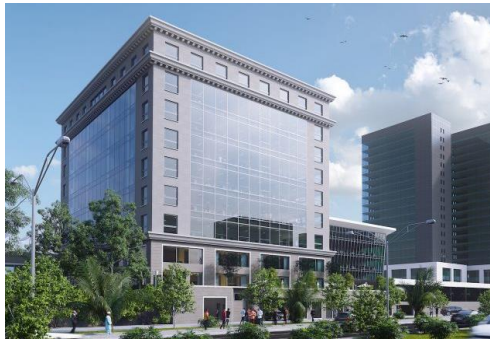
Figure 147 Image of Delta Chambers, Nairobi. Source: Delta-Chambers-750x450.jpg (750x450) (towercost.co.ke)
