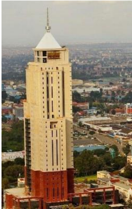
Figure 9 Image showing UAP Old Mutual Building in Upper hill Nairobi. Source: upp2-252x400.jpg (252x400) (biggestkaka.co.ke)
