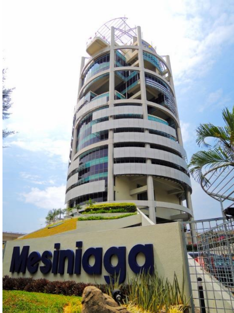
Figure 60 Image showing Ken Yeang's Bioclimatic building; Menara Mesiniaga.
