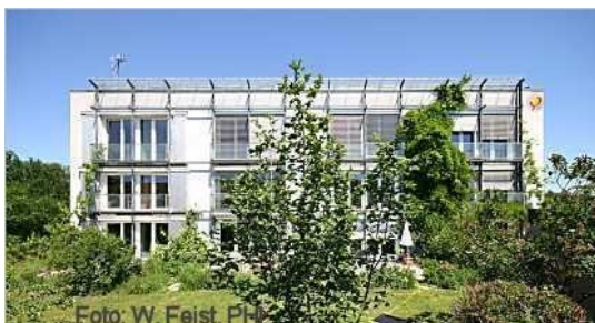
Figure 28 Image showing Wolfgang Feist and Bo Adamson created a sketch of the "Passive House." Source: passivhaus_kranichstein_sued.jpg (415×222) ( passipedia.org )
