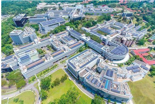
Figure 48 Image showing installed solar panels on the rooftop of the NTU Campus Building in Singapore.
