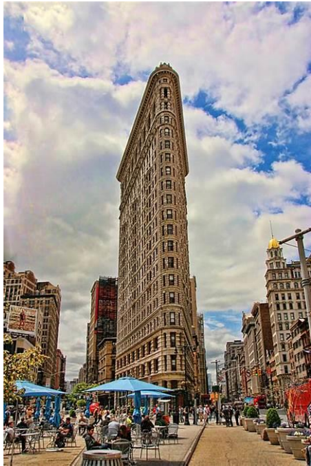
Figure 34 Image showing Flatiron Building in the USA among the first buildings to employ HVAC systems. Source: OIP.kA-N9XIXPIRicwKypAN1xwHaLI (466×700) (bing.com)
