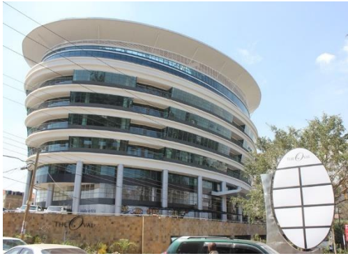
Figure 111 Image of Oval Building in Westland's Nairobi. Source; R.b0ee427c355a4ff17850be24aad140b9 (826×600) (bing.com)
