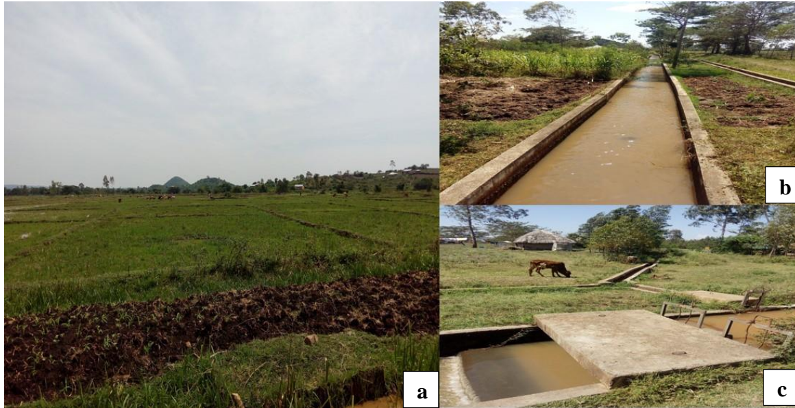
Fig. 3. 2 The images indicate the (a) flood, (b) and (c) concrete canal irrigation systems in the irrigated zone in Homa Bay in western Kenya.
