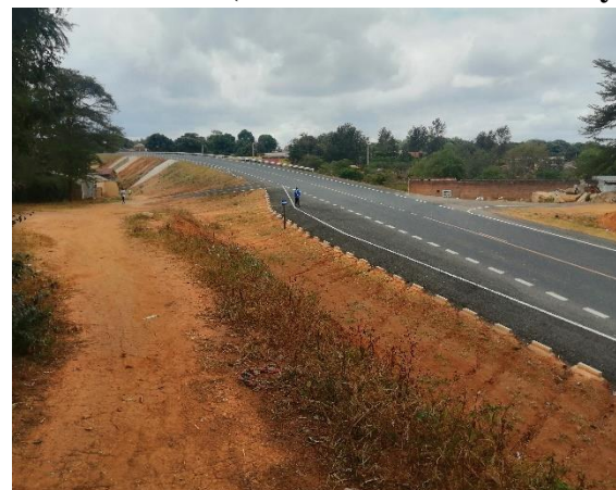
Plate 6: New A9 (New Kibwezi-Kitui-Kanyonyo Road)
