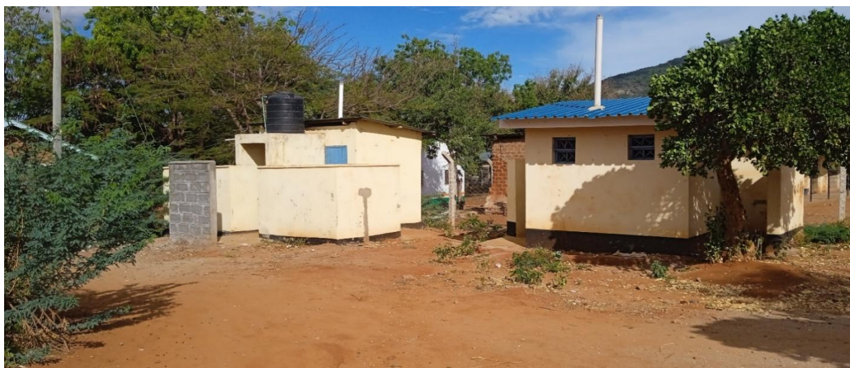
Figure 5.3 Public Toilet & Bath Facilities
