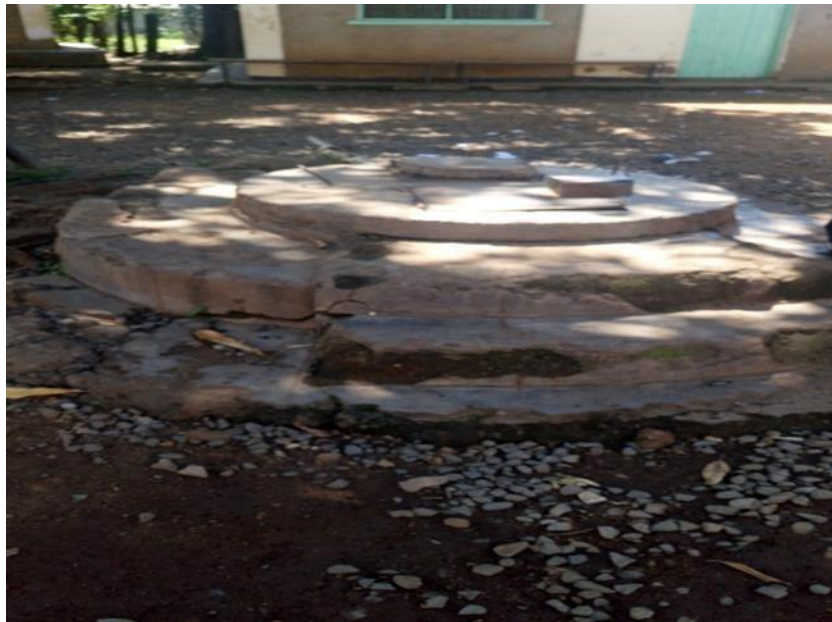
Figure 7.5: St. Edward Catholic's Church well
