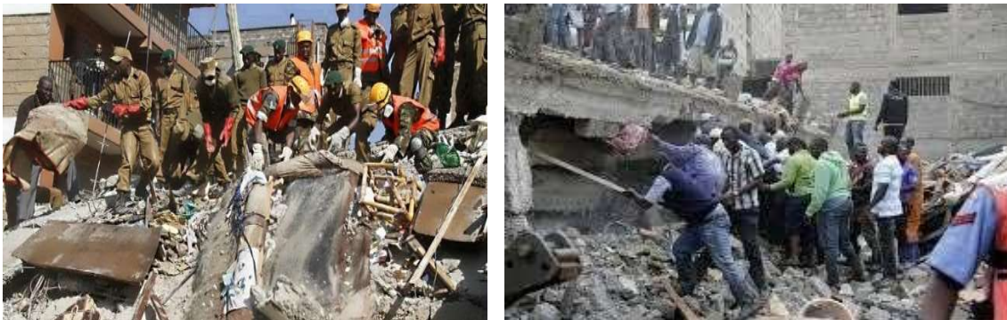
Plate 1.1: Rescue operation in collapsed buildings in Nairobi Source; (NCA, 2021).
