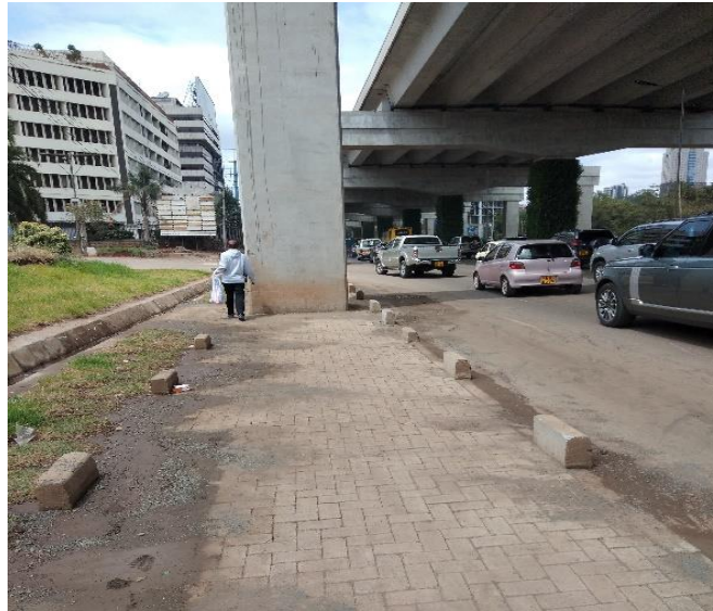
Plate 3-5: Obstruction to Pedestrians Walking along Uhuru Highway, Source: Author, (2022)
