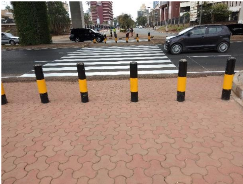
Plate 4-4: Crash barriers installed at midblock crossing. Source: Author, 2023
