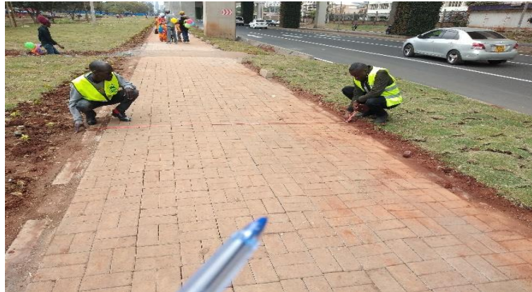
Plate 3-1: Road geometric features along Uhuru Highway, Source: Author, (2022)
