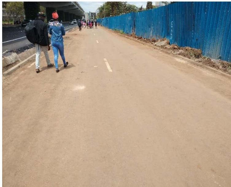
Plate 3-6: Ongoing Construction Activities near Uhuru Highway, Source: Author, (2022)
