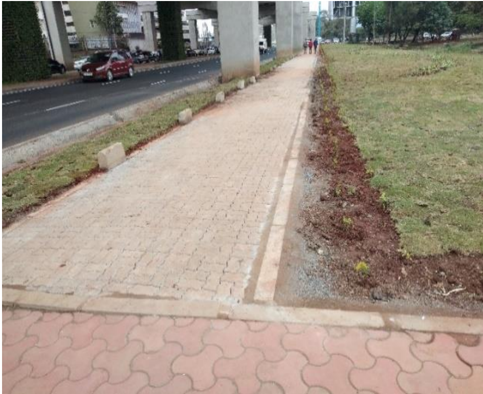
Plate 4-5: Improved pedestrian walkway along Uhuru Highway. Source: Author, 2023
