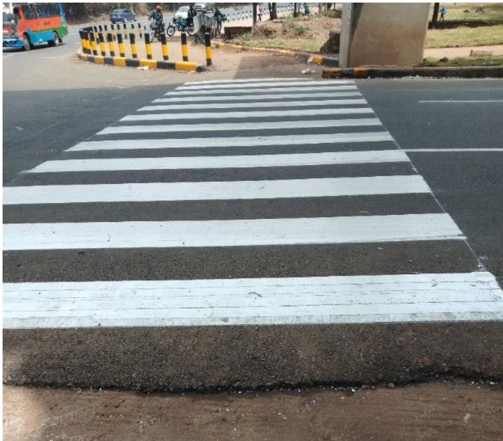
Plate 4-6: Pavement markings installed at crossings near roundabouts. Source: Author, 2023
