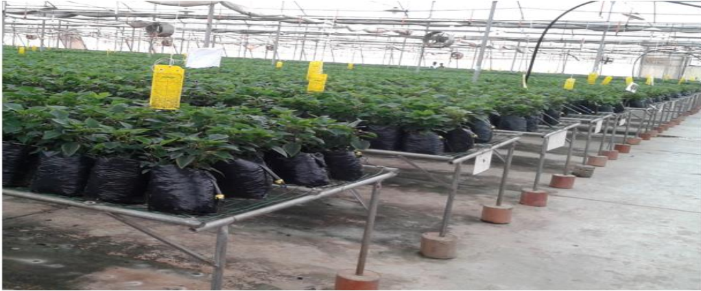
Figure 4.2: Steel benches supported with steel pillars on a concrete floor.
