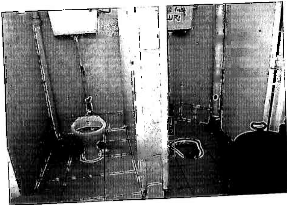
Plate 04;- Clean, tiled floors and walls inside toilets in privately-run toilet block at the City Market. The high English type toilet on the left is for the disabled and aged while the squatting type on the right is for ordinary users
