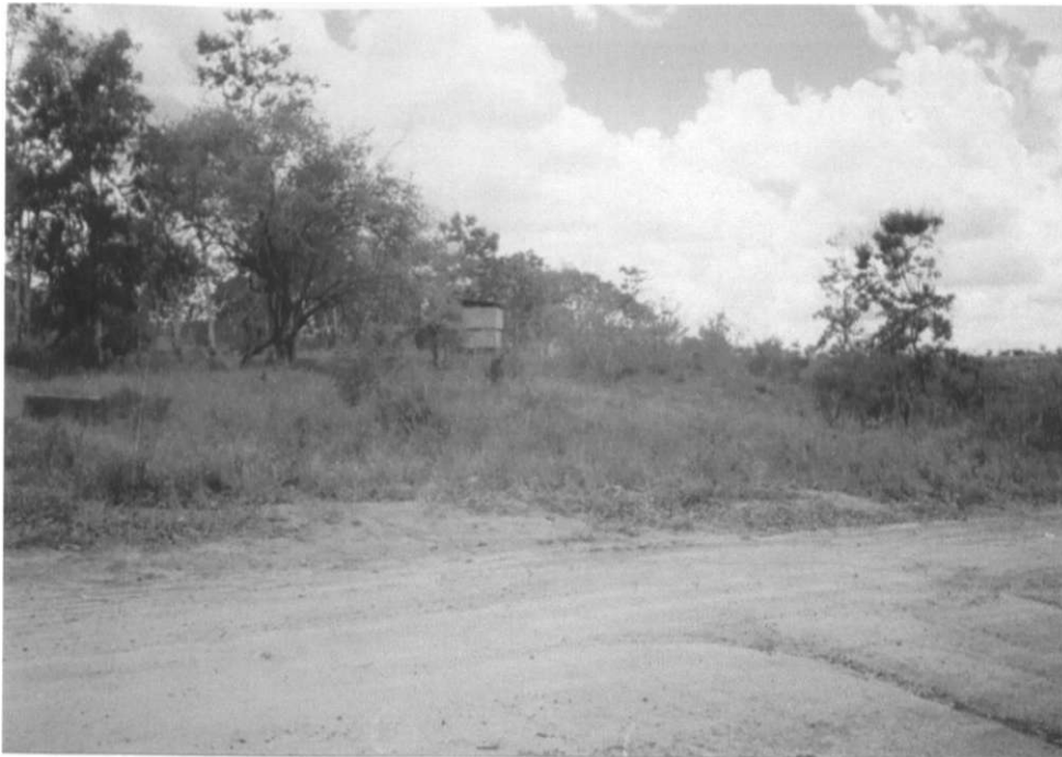
Plate 9. This is what remains of the Kibaoni water kiosk after the collapse of the project some seven years ago.
