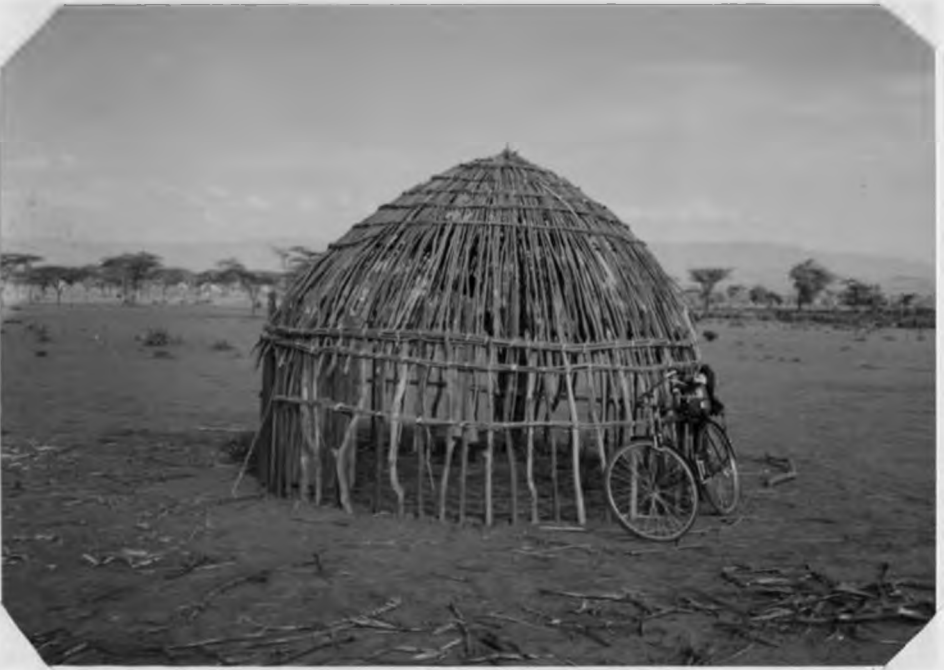
Plate 4.4: "Manyatta" construction: This consumes quite a substantial amount of biological resources (Author).
