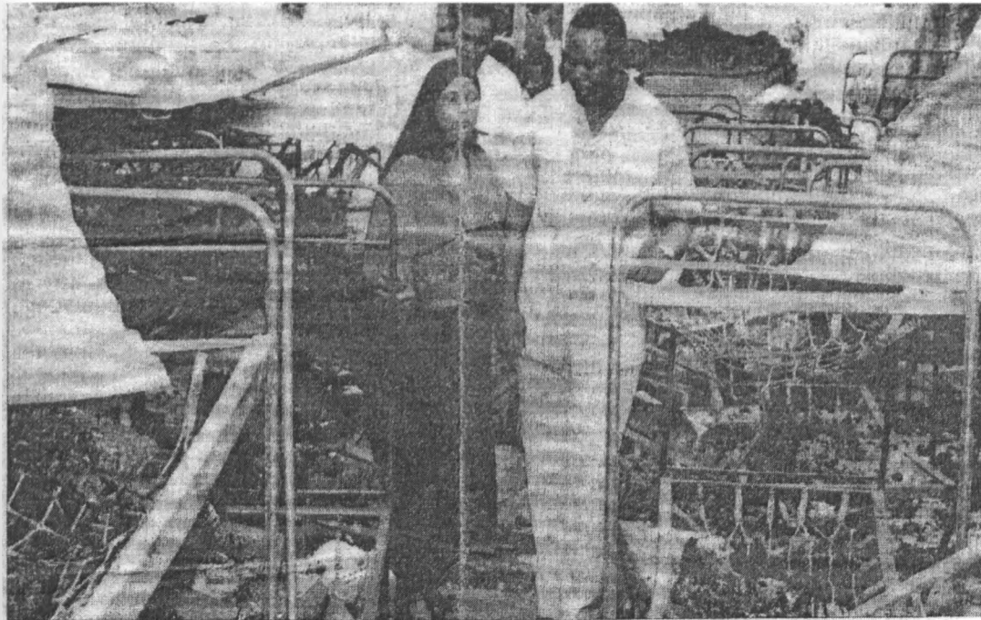
A dormitory in one of the Kenyan schools destroyed by a fire outbreak
