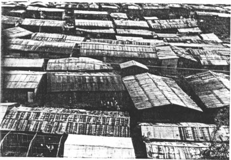
Plate 1: Mathare Valley. (This part of mathare valley in Nairobi demonstrates the poor conditions under which many of the city residents are living).
