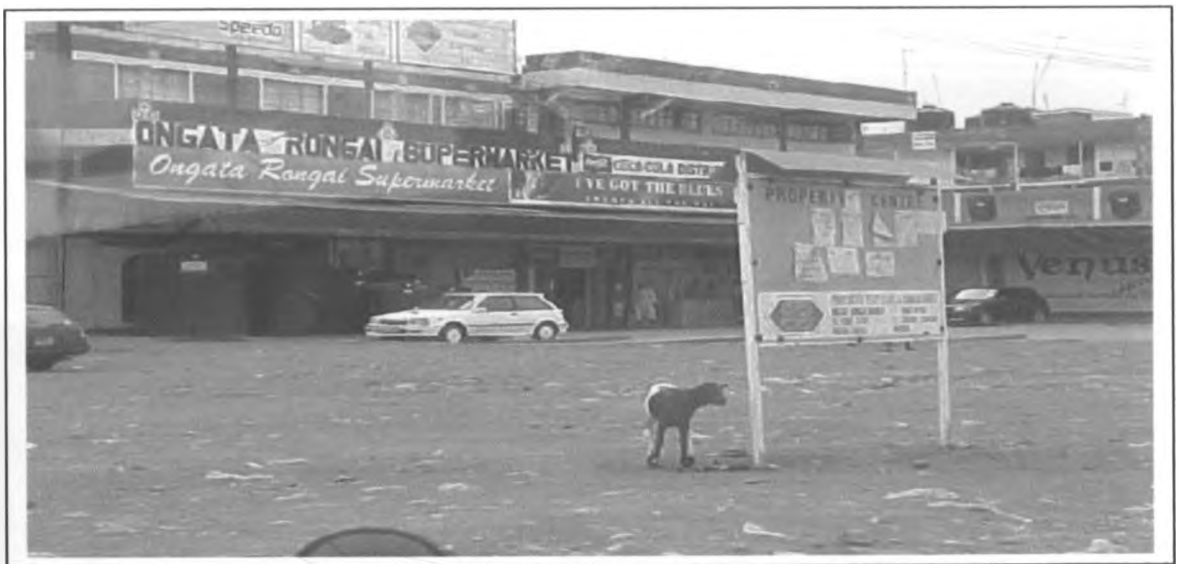
Fig. 15 – Showing a commercial complex in Ongata Rongai
