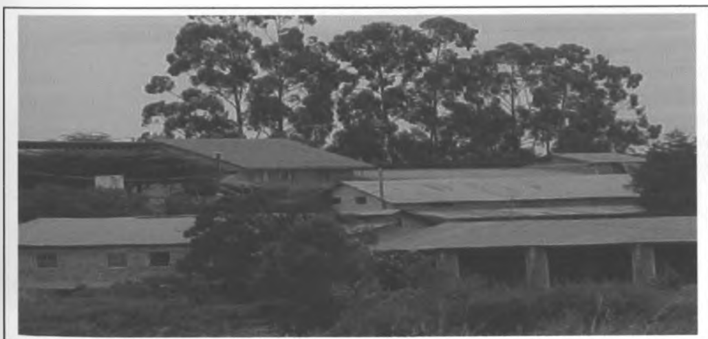
Fig 10 – Built-up Area bordering Athi River
