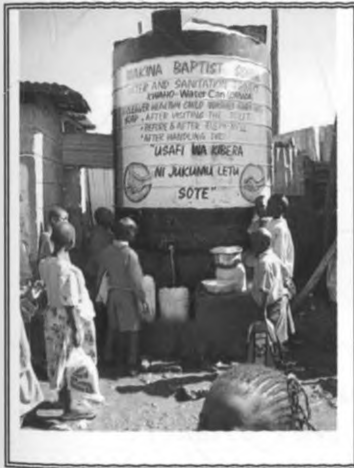
Photo 4.4: A communal water point in Kibera (Source: Fieldwork)
