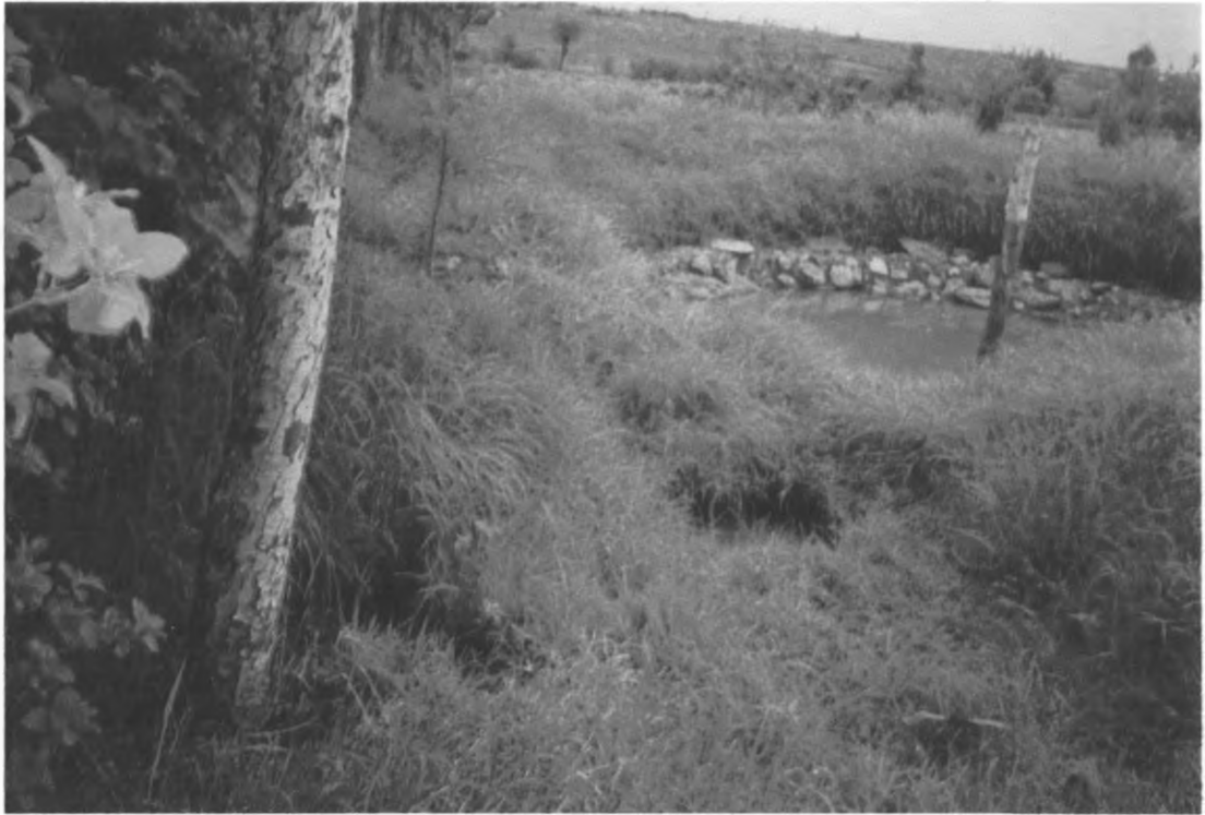
Plate 4.3: Masonry lined water pan showing a grassed inlet and siltation pool
