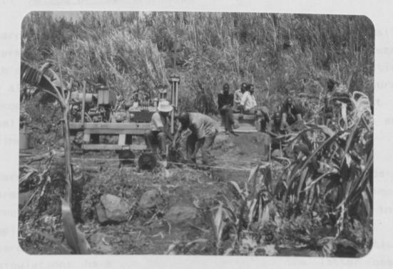
Plate 4.4 Core drilling in progress at BH2. Note V.E.S. S17 being conducted next to the borehole. The spread is along the flat valley bottom with the steep rise on the right abutment seen on the background.
