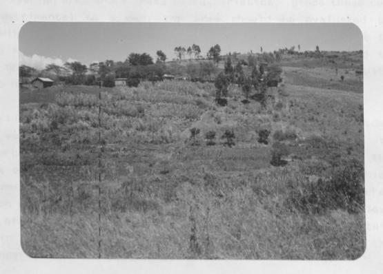
Plate 1.4 Photograph of the dam site taken from BH5 facing north. The dam-axis is indicated with the dashed line. Note the exposed boulderly basalts covering the right abutment. The ridge rises to 100 m above the elevation of the valley at the far horizon next to Nairobi-Kiserian road.
