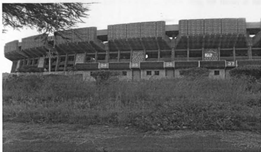
Photograph: 5.6 Main Stadium Compound near the Gates
