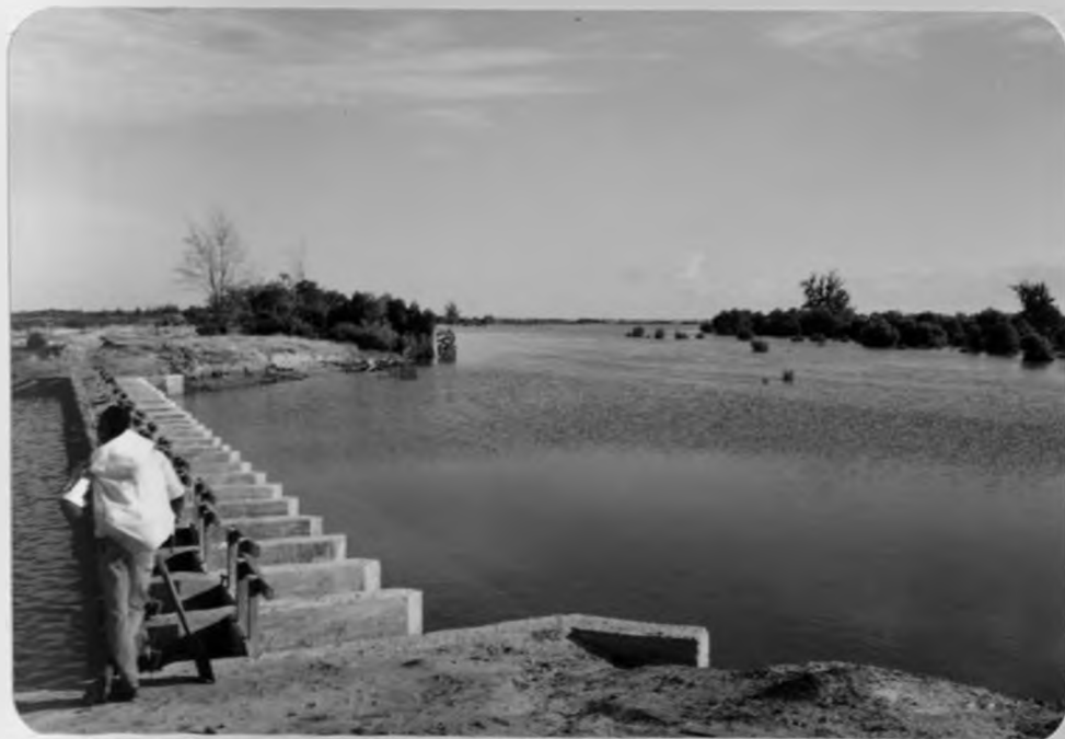
Plate 29. A lagoon behind Robinson Island. In the left margin of the photograph are sluice gates leading to salat extraction ponds.
