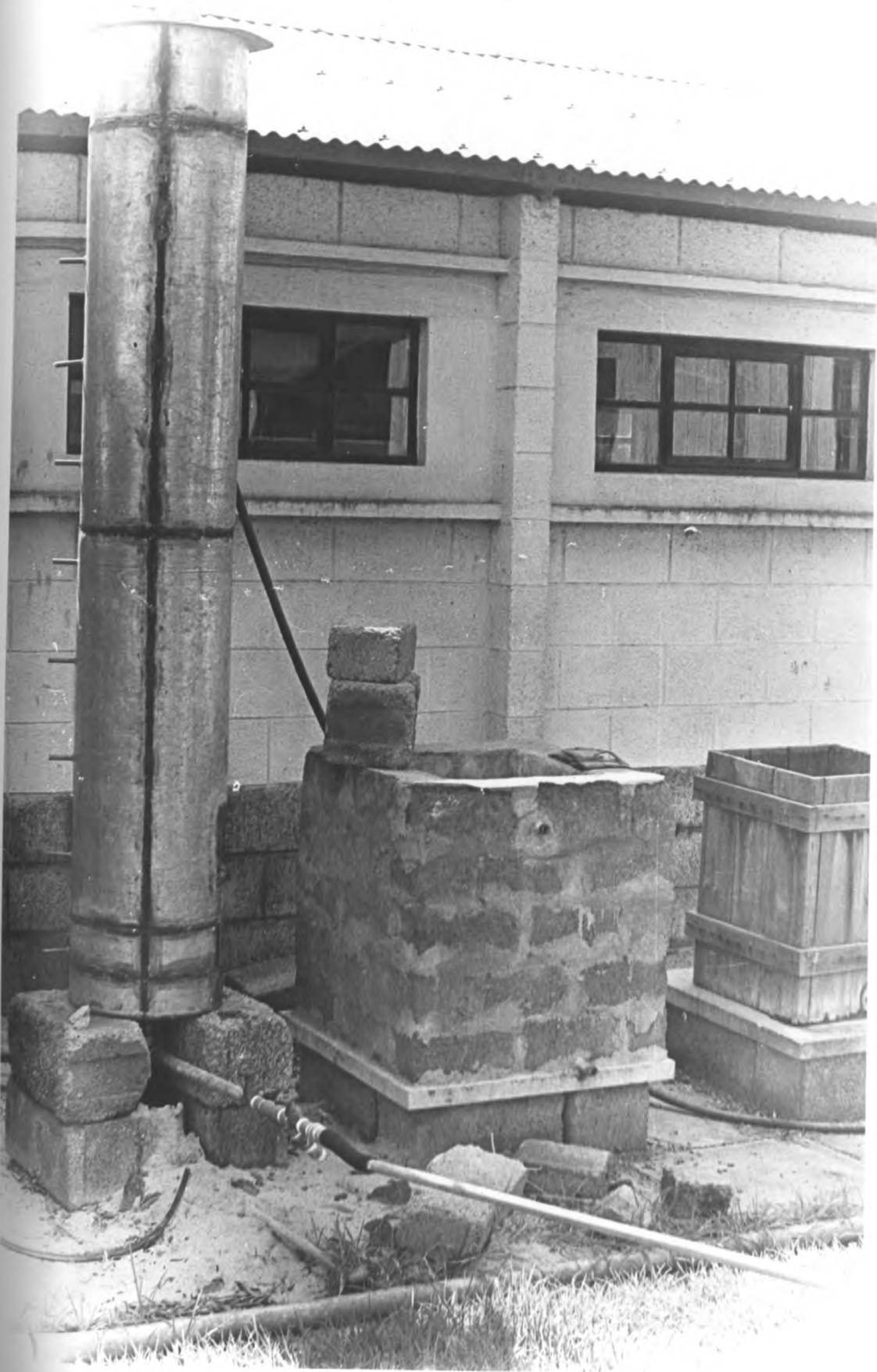
Plate 7C Filter in position
