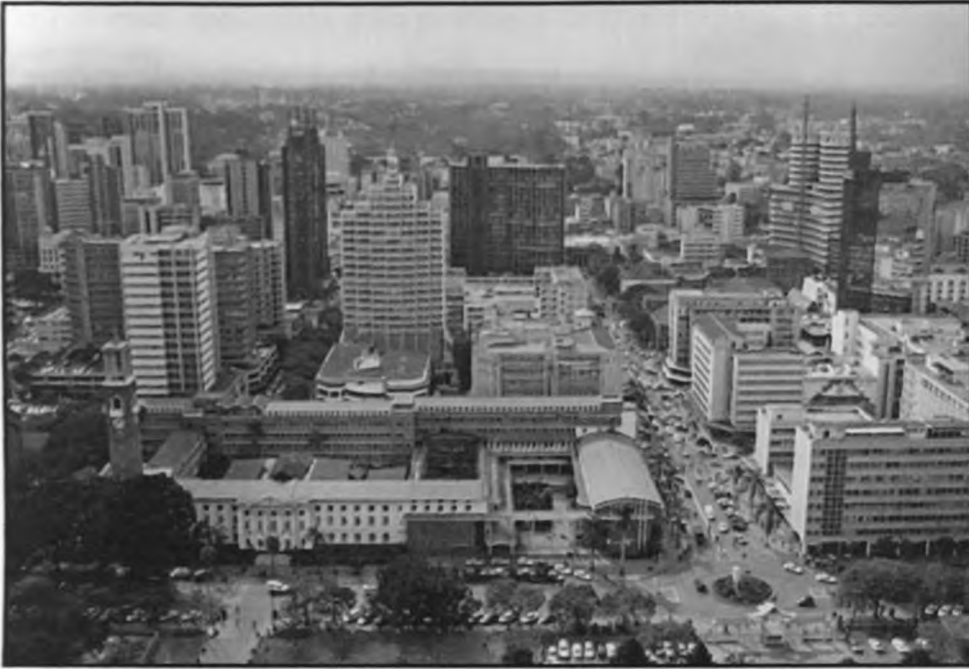
Photo 1.1: Picture of the CBD of Nairobi City (notice the high skyline)
