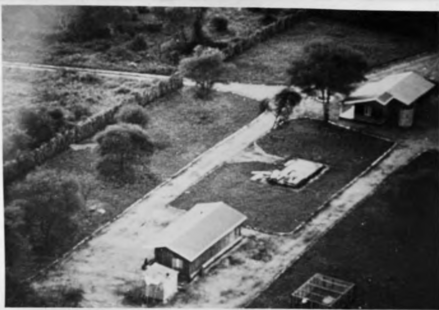
Plate 1 Gas Division Field Camp at Tenet
