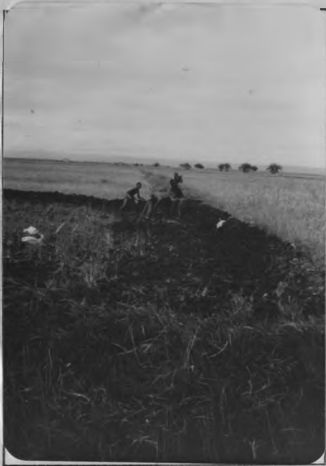
PHOTO 5: Backfill after Being Placed in Trench
