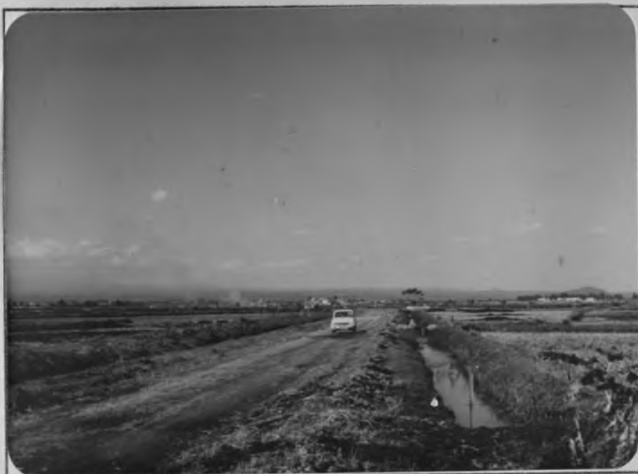
PHOTO 6: Intervening Section of the Canal Filled with Water (Canal Seepage Experiment)
