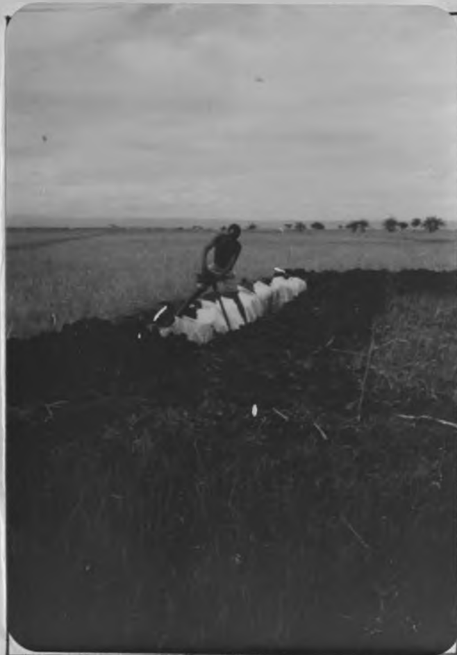
PHOTO 4: Backfill Being Placed Around the Polythene Sheet
