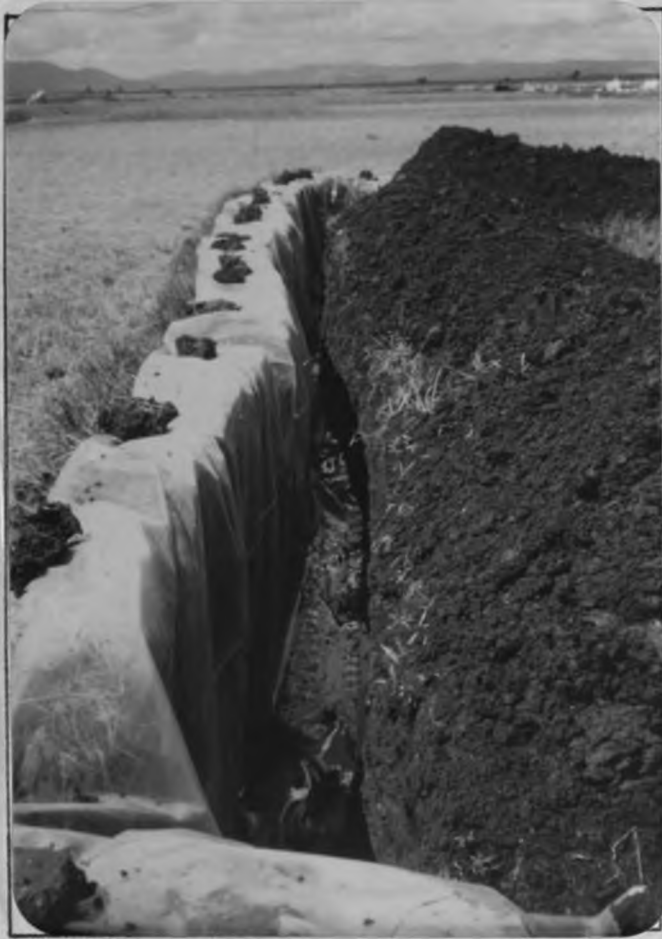
PHOTO 3: Polythene Sheet Lined Around the Trench
