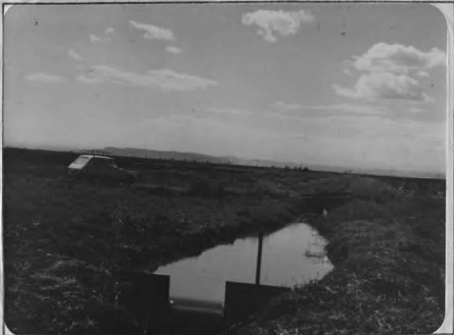
PHOTO 1: Rectangular Weir Located at the Outlet of H2
