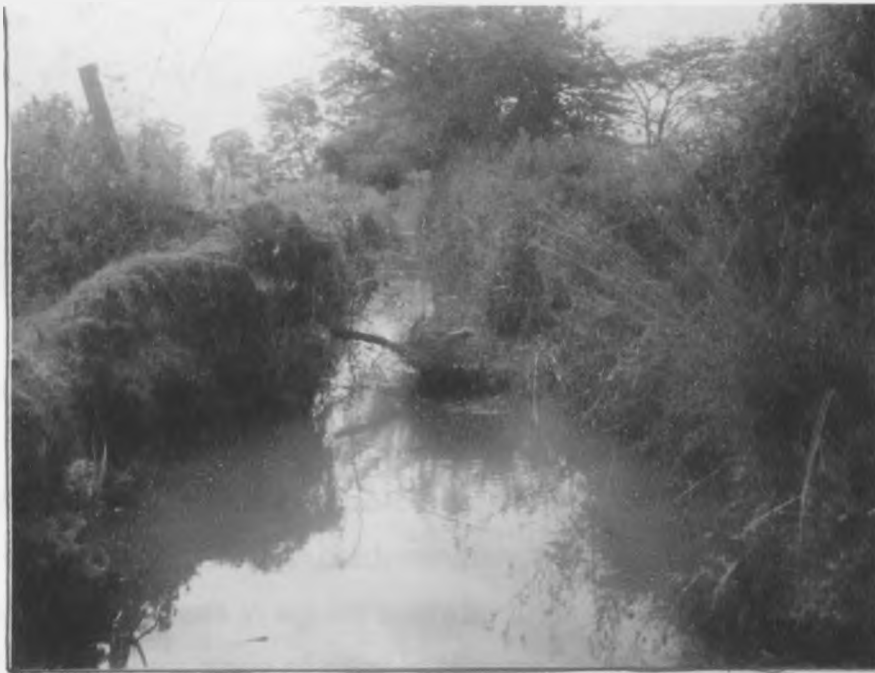
Plate 4: A damaged section of main furrow in Thome scheme
