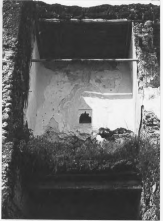
34 House in Mkomani- Ngao showing mwandi
