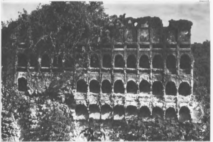
38 House in Shella- Ruined zidaka
