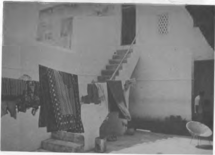
31 House in Mkomani- Kiwanda
