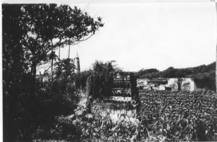
37 House in Shella- Ruined zidaka
