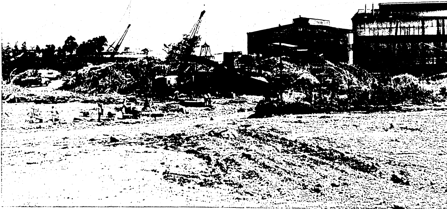
PLATE 11 Muhoroni factory. One of the two 3 major factories in the Sugar-belt.
