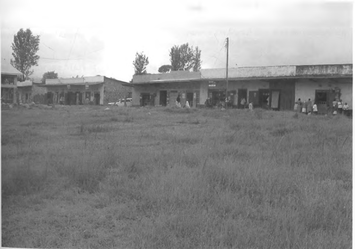
Ntharene Old Market Centre: Background shows the shopping centre. The foreground is an open space set aside for an open – air market, but instead open – air market business is conducted on the road reserve.
