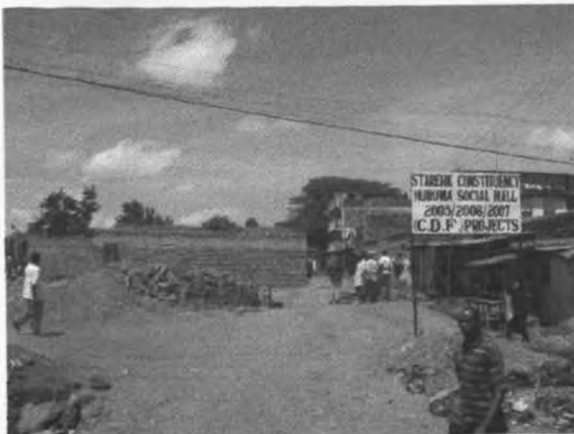
Plate 4.23 Construction of Community Centre
