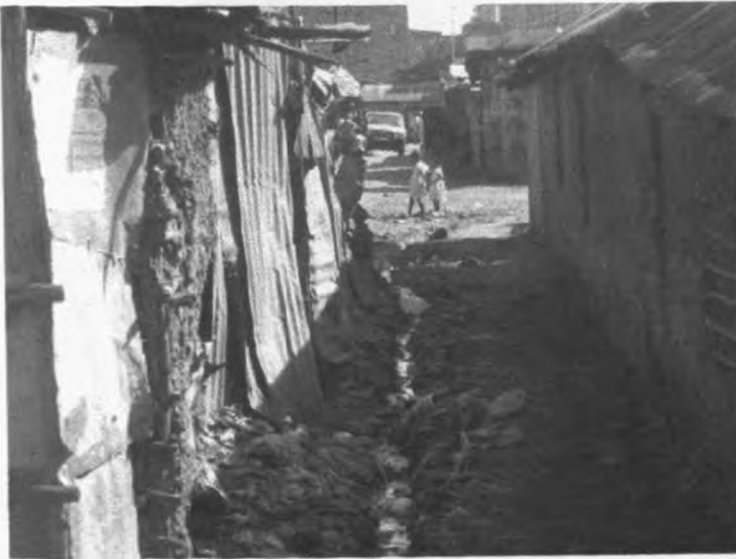
Plate 4.28 Open Drain and Rubbish in Alley
