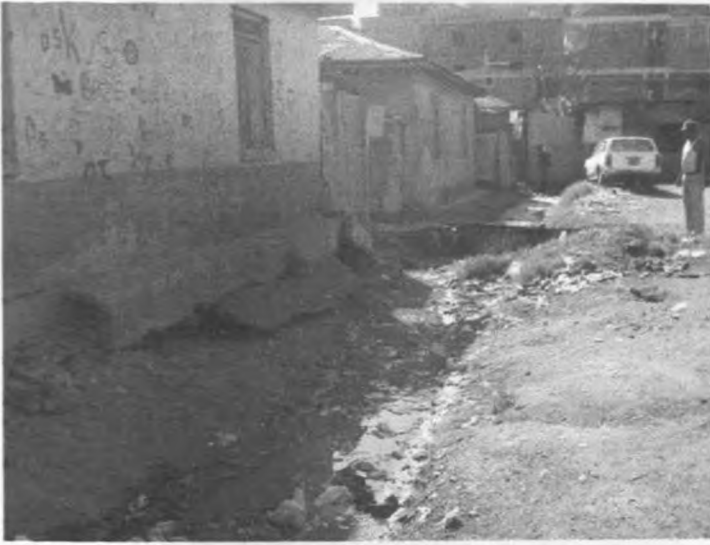
Plate 4. 27 Open Road drain carrying human waste
