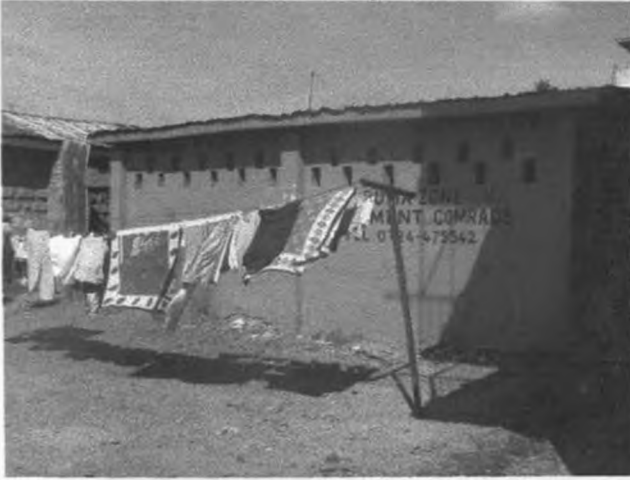
Plate 4.24 Converted Sanitary Block.
