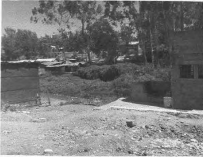
Plate 3.2 Construction next to the river
