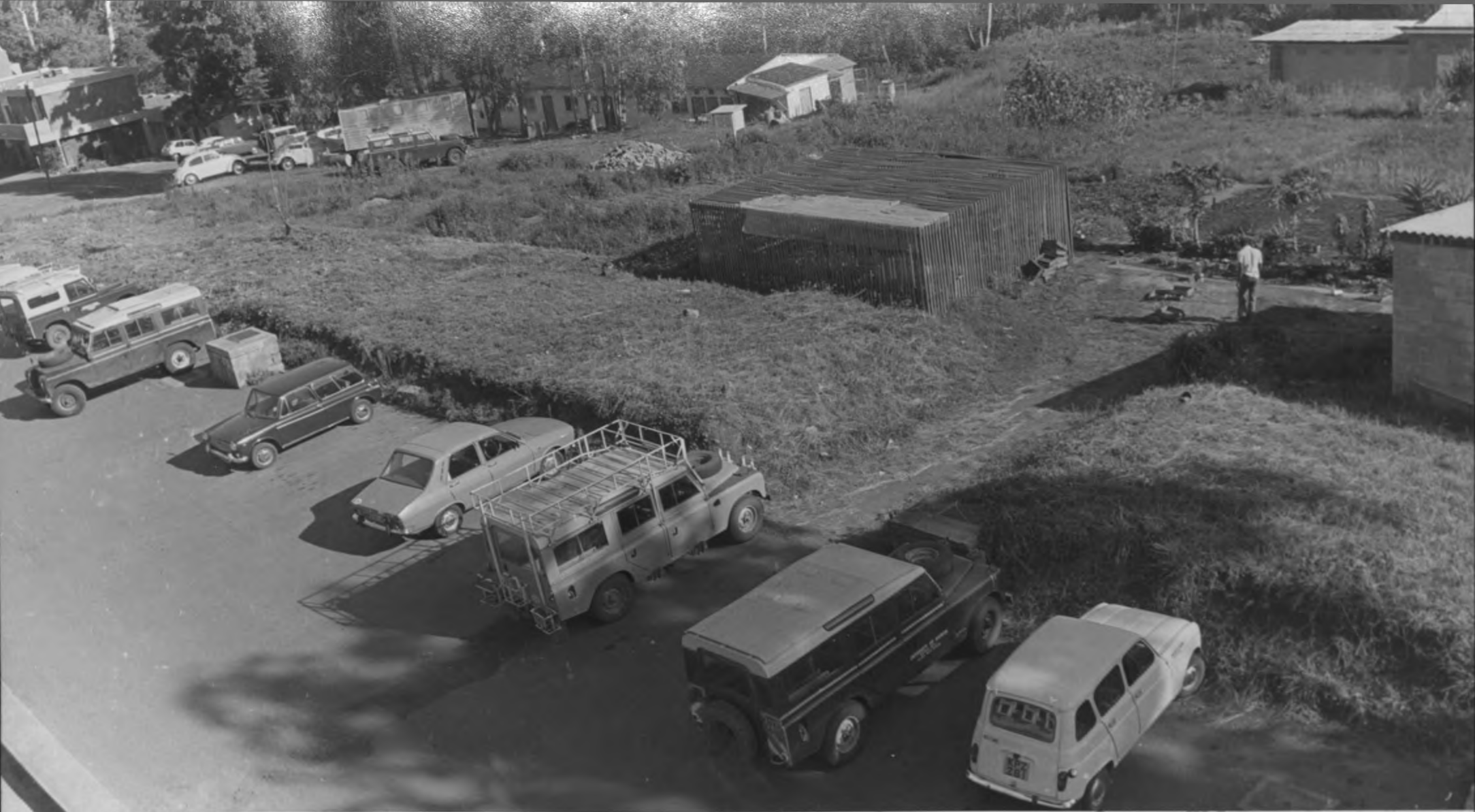
PHOTO 1: Part of Site as seen from the Zoology/Potany Building. I.C.I.P.E. new buildings seen in part on the left. Old I.C.I.P.E. seen in the background to be demolished.
