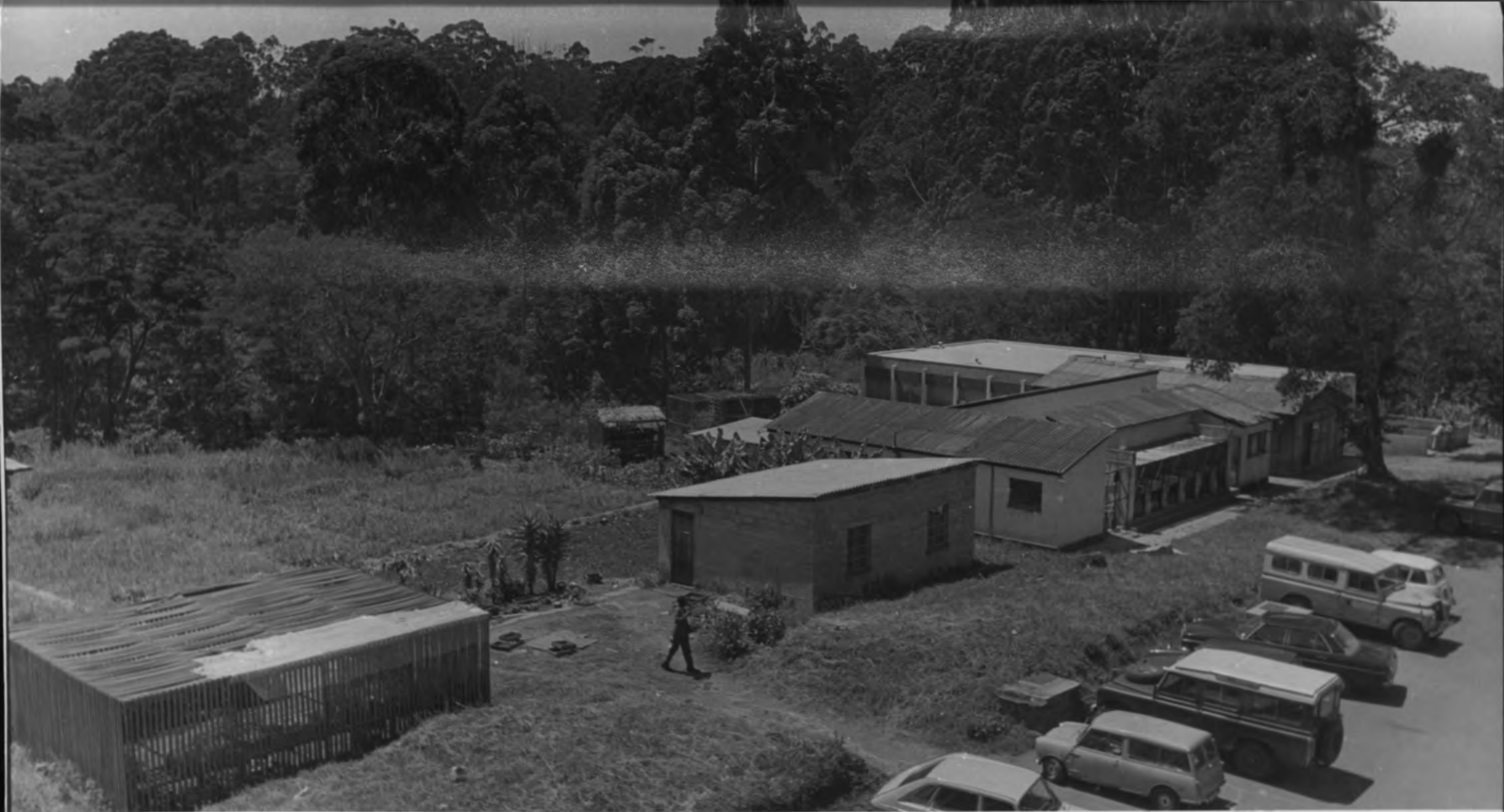
PHOTO II: Another part with Gecaga Institute in the background on the right. Other structures to be demolished
