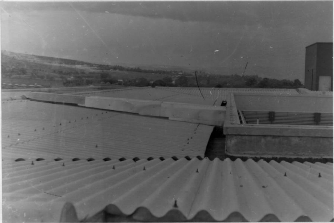
PLATE I FALSE ROOF OVER A FLAT ROOFED BUILDING
