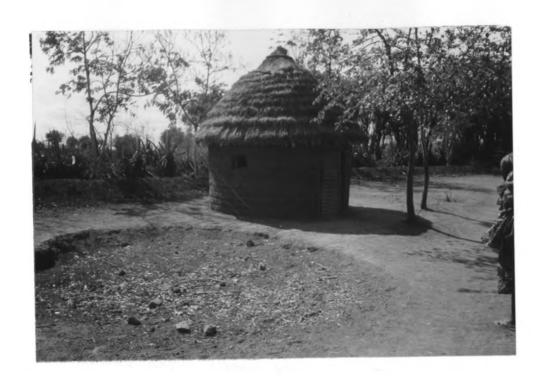
Plate 4.1: Traditional round house made of mud brick walls and a thatched roof.
