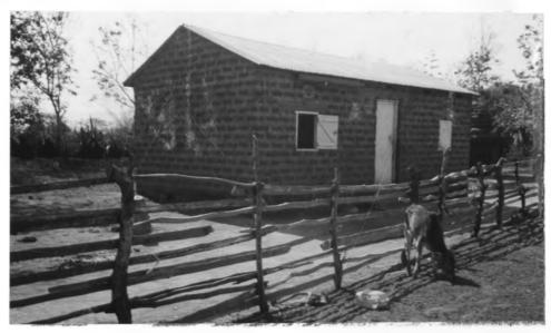
Plate 4.3: Rectangular house made of fired brick walls and a corrugated iron sheet roof.
