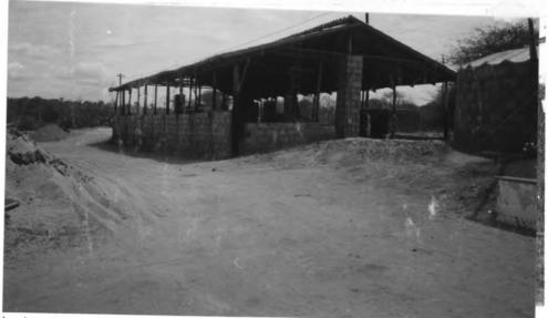
Plate 4.4: House constructed with concrete block walls and a corrugated iron sheet roof
