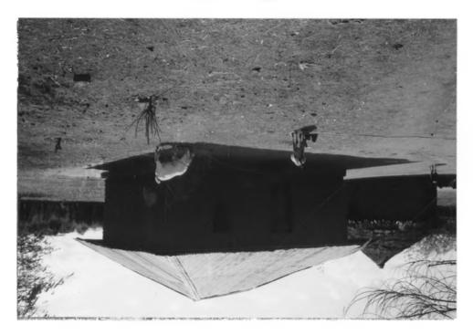
Plate 4.2: Rectangular house made of mud brick walls and a corrugated iron sheet roof.
