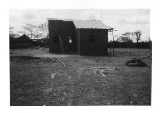
Plate 4.5: House constructed with concrete block/natural stone walls and a tile roof. These designs are mainly constructed by the Kauwi Muugano project
