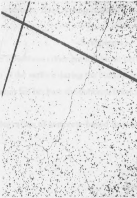
Photos 1, 2 & 3 Cracking of dense, in situ, floor finishes.
