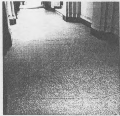
Photos 1, 2 & 3 Cracking of dense, in situ, floor finishes.
