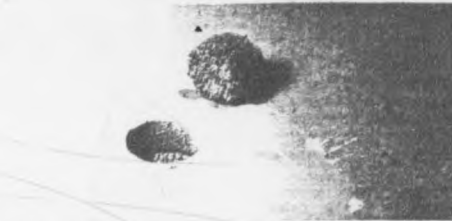
Photos 4 & 5 Cores drilled from a granolithic floor topping showing poor compaction and a high percentage of voids.
