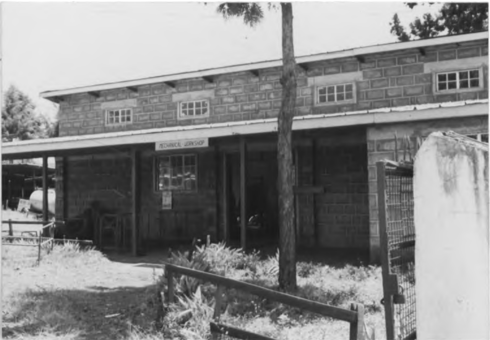
Plate 4.6: Mechanical Workshop at Kirwara. It operates at a very low level.
