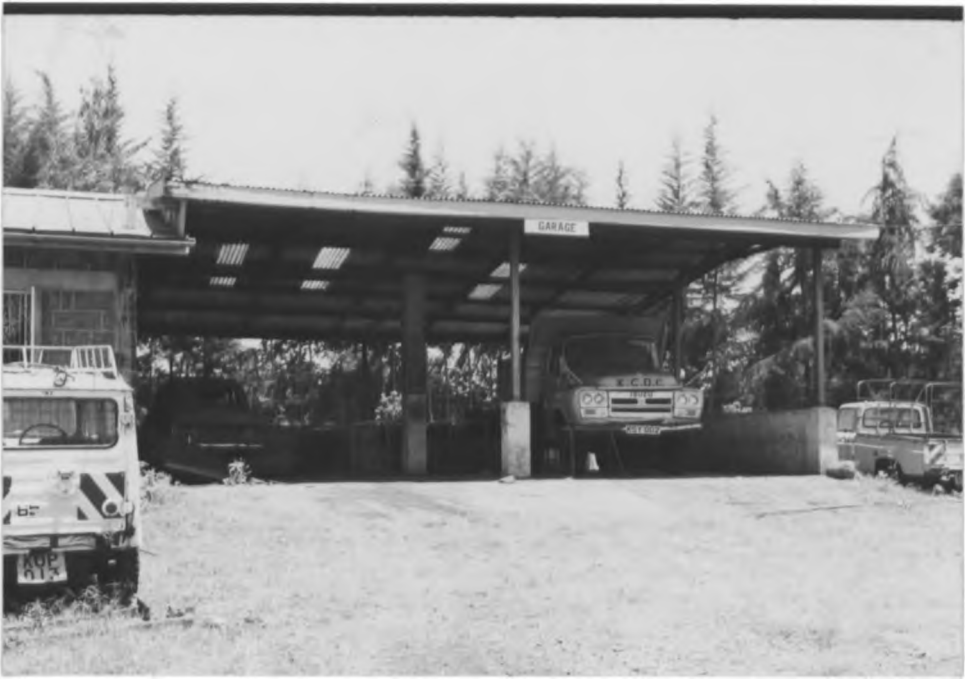
Plate 4.5. This is what used to be a garage. It is no longer operational.
