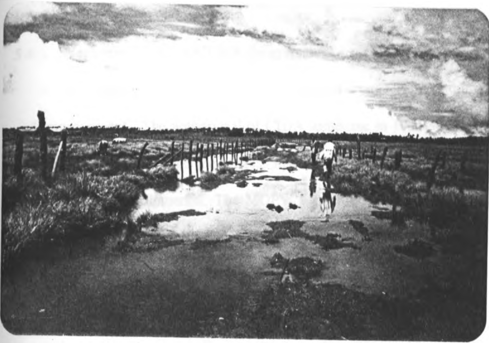
Plate 10: A Rural Access Road Completely Flooded
