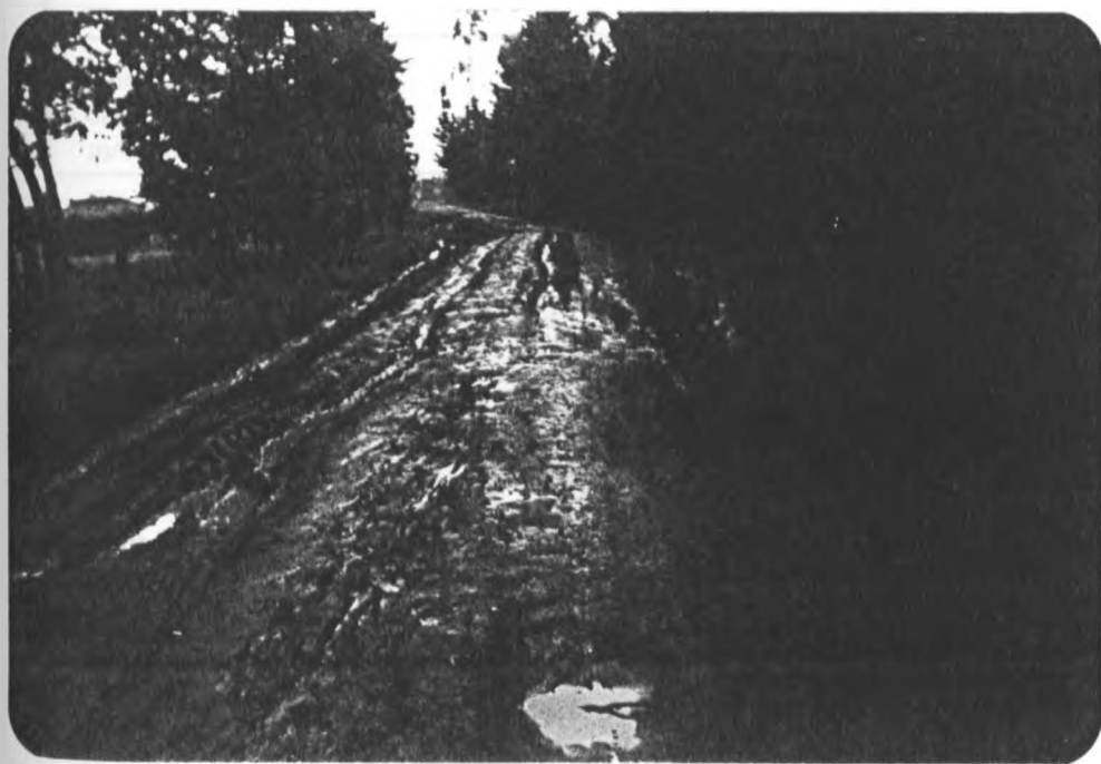
Plate 12: Most Access Roads Are Not Yet Gravelled, Hence, Impassable, during the wet seasons.
