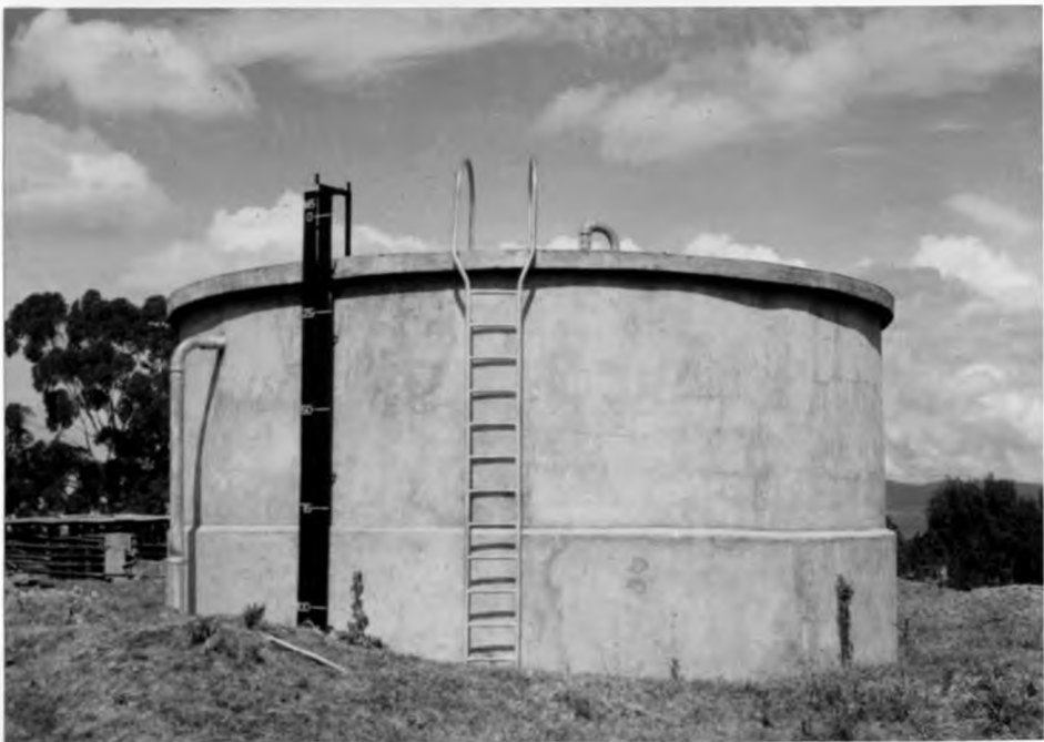
Plate 4-4: Water Reservoir at Taitta Toweett
