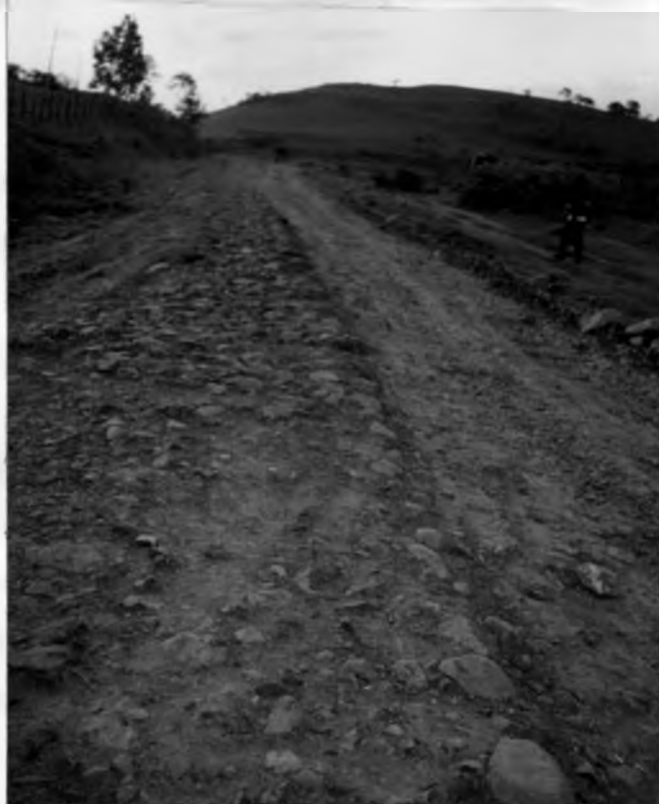
Plate 4-9: Rough Road Surface (Note the presence of rock protrusion and gullies created by rain water).
