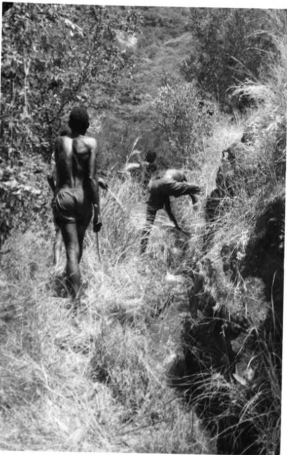
Plate 4.3: The clearing of Furrow sides - Kapterik.
