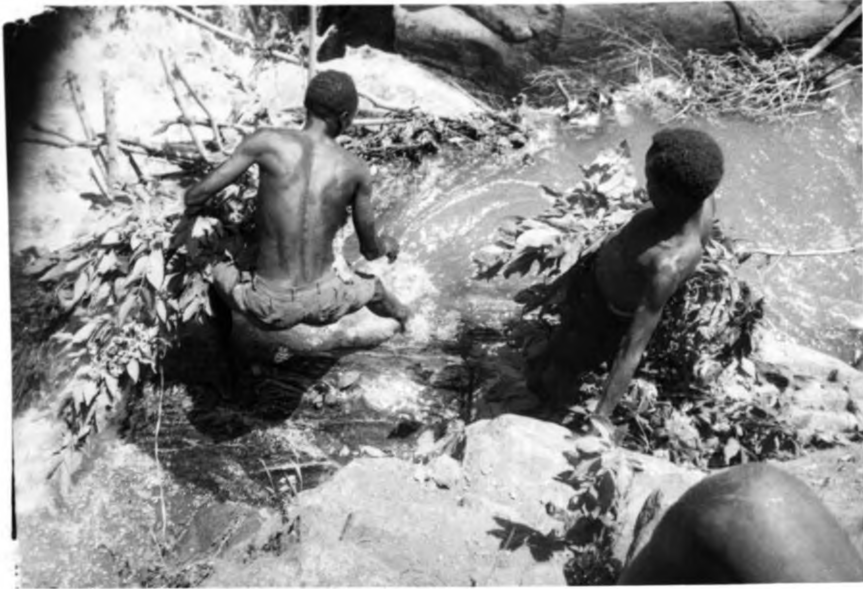
Plate 4.2: The Reinforcement of an Indigenous Furrow intake - Kapterik Furrow.
