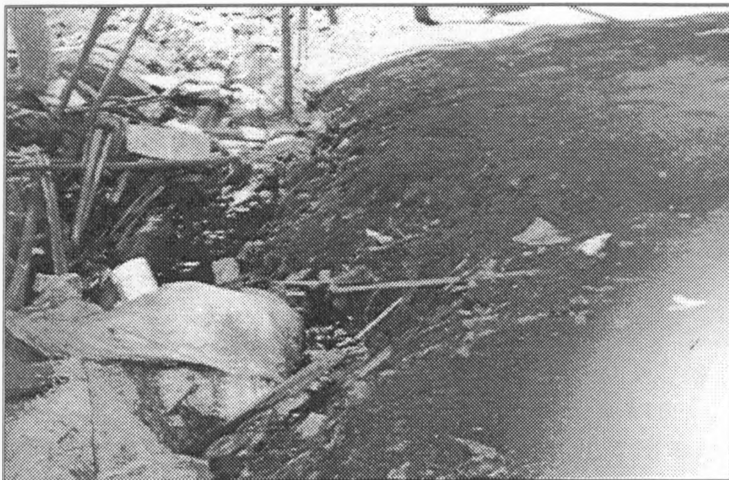
Plate 5-2 Poor Drainage Systems within Githurai Market.
