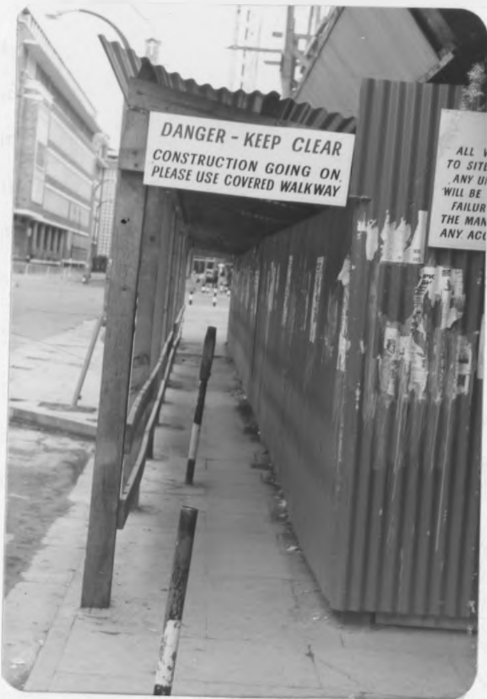
PLATE 6: A properly constructed gangway. A necessity for all sites in the city centre. Note the warning poster. This photograph was taken at City Centre, Nairobi, in 1987.
