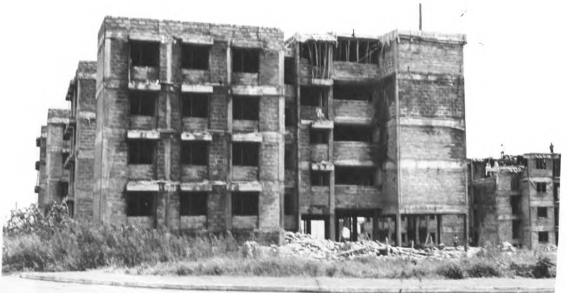
PLATE No.2: Huruma Rental Scheme when it was under construction
