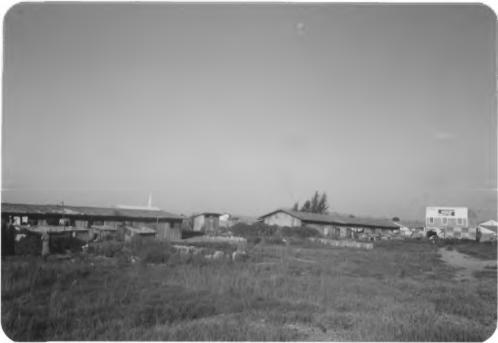
Plate 5: Semi-permanent houses built for those members working in the factory
