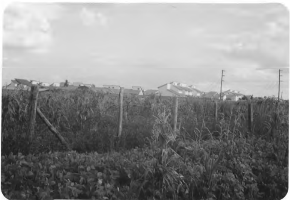
Plate 8: Komarock Housing Estate (phase 1) where the group's sisal-cement roofing tiles were used.
