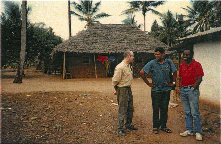
Plate 3.1. Study area showing a house made of mud walls and roofed with dried coconut leaves ( makuti ).
