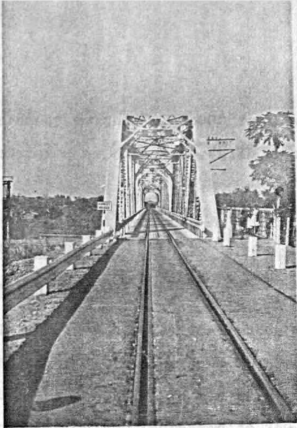
Plate 5: Newly built rail-road bridge at Chiromo.
