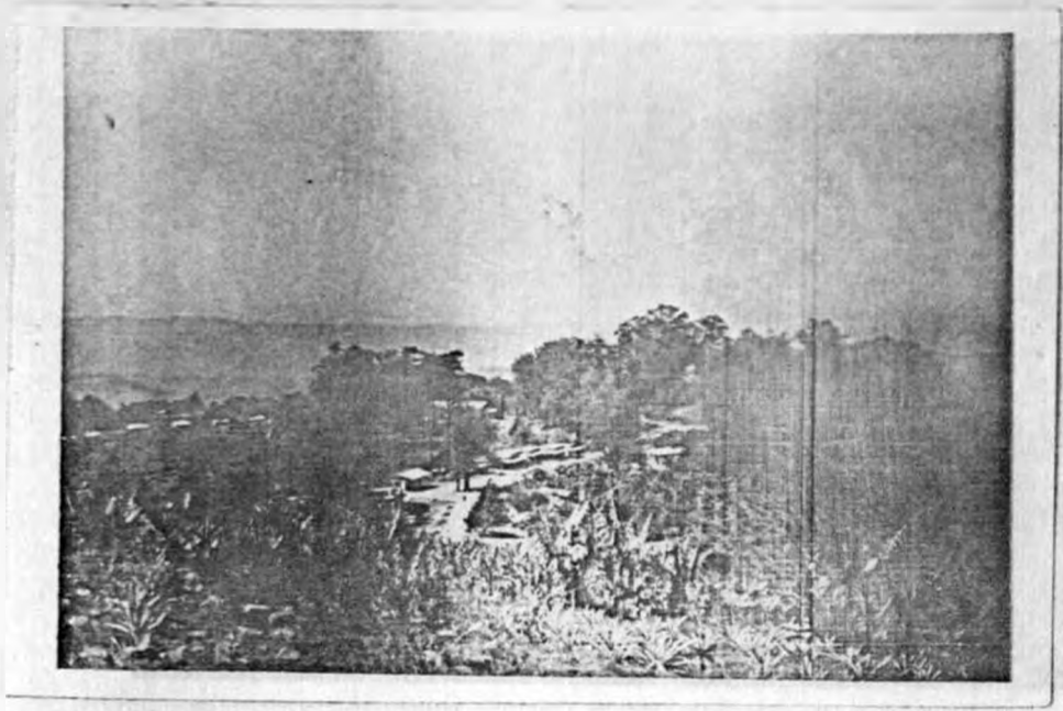
Plate 9: Looking down Thekerani Rural Growth Centre from a nearby hilltop.
