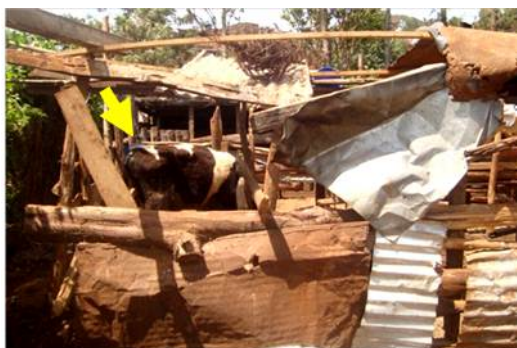
Figure 11. Collapsed iron sheet roof and sides in one of the zero-grazing units evaluated. Both the roof and side timber are broken and collapsing. Yet cows are still housed inside (arrow).
